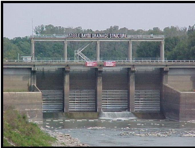
Steele Bayou Drainage Structure
